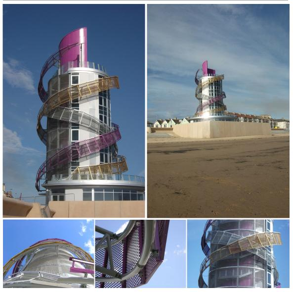
Broadway Expanded Metal and Coburg 12-12-12 Architectural Wire Mesh installed at Redcar Vertical Pier as part of a wider seafront regeneration project.
