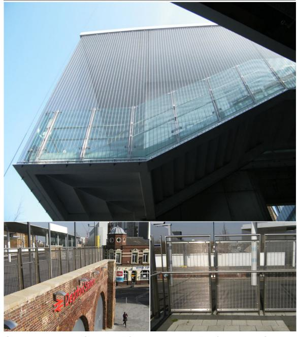
Gladstone 80/10 and Gladstone PC 80/10 installed at Deptford Railway Station, London. Gladstone 80/10 was installed using the cable mesh tension system around the stair tower and Gladstone PC 80/10 was used as balustrading around the station and cycle store.
